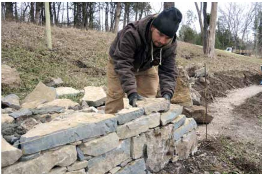
A worker from the Parke Company lays dry-stack stone to expand the rock wall that runs along the hill beside the City Hall driveway. The wall follows the contour of the old Brentwood Pike, now Old Hickory Boulevard.
